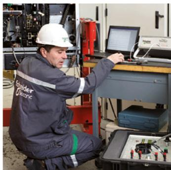
Regular diagnosis of electric and kinematic performance of LV circuit breakers is delivered with the Advanced Manufacturer Maintenance program. This solution brings the end user the following benefits:
